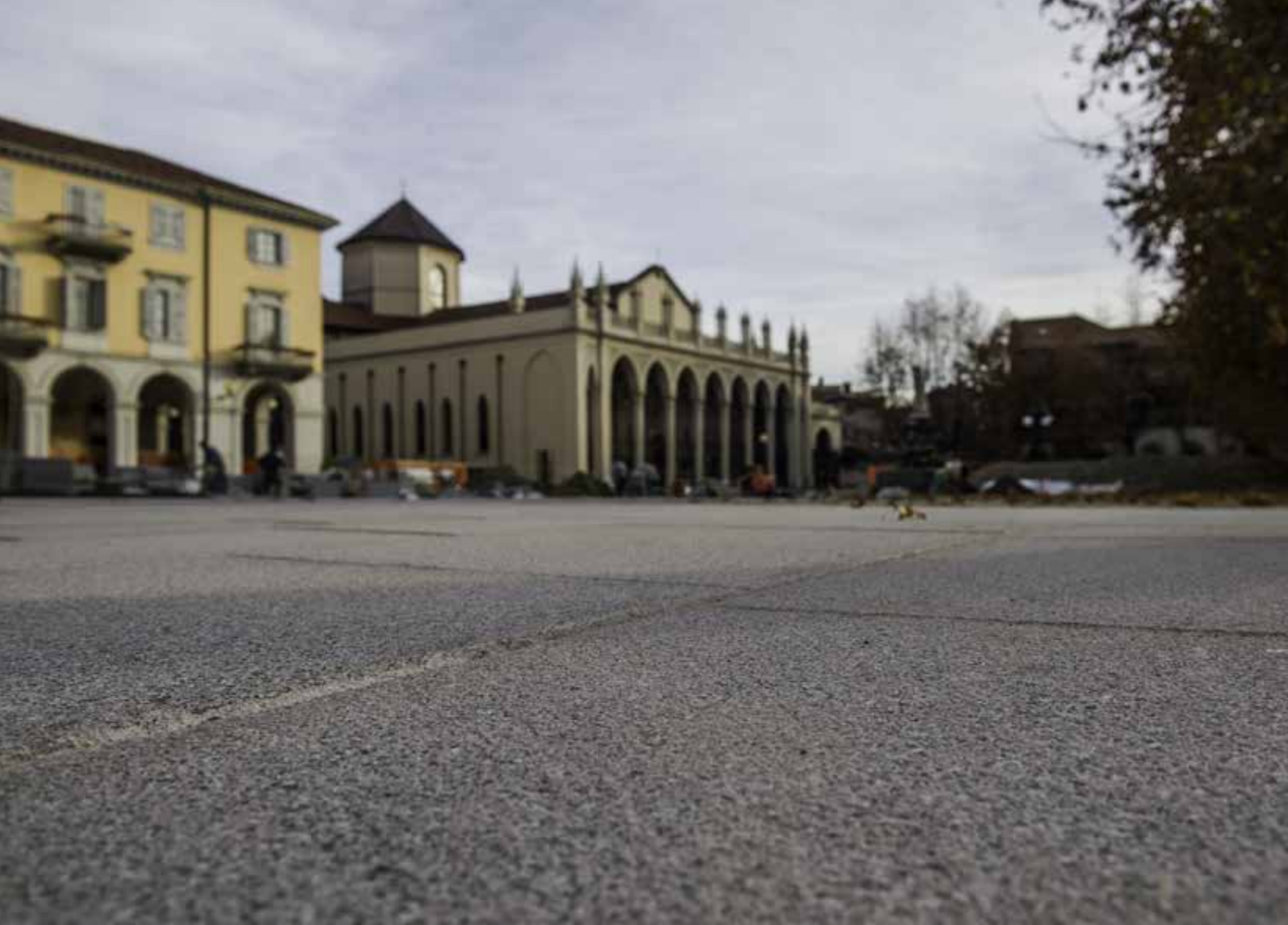
Scala in Luserna granigliata Scratched Luserna staircase
